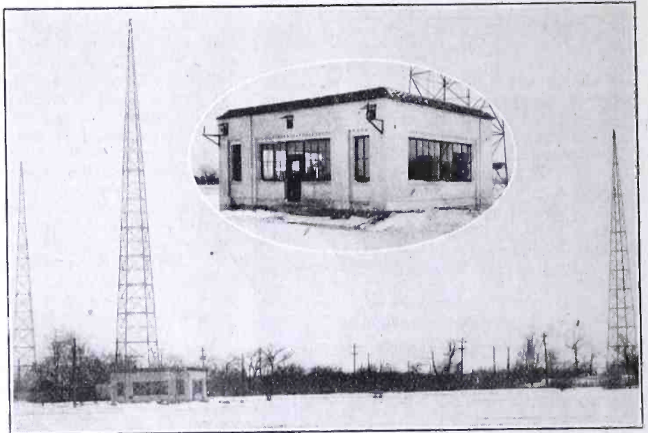
Towers and Building at KDEN
