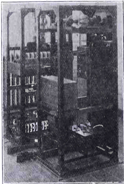
Transmitting and Rectifying Equipment at KDEN
